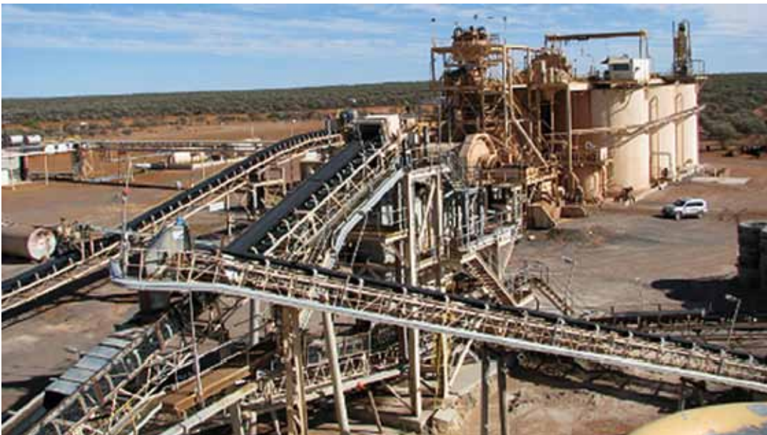
Figure 1 Kirkalocka Gold Processing Plant
